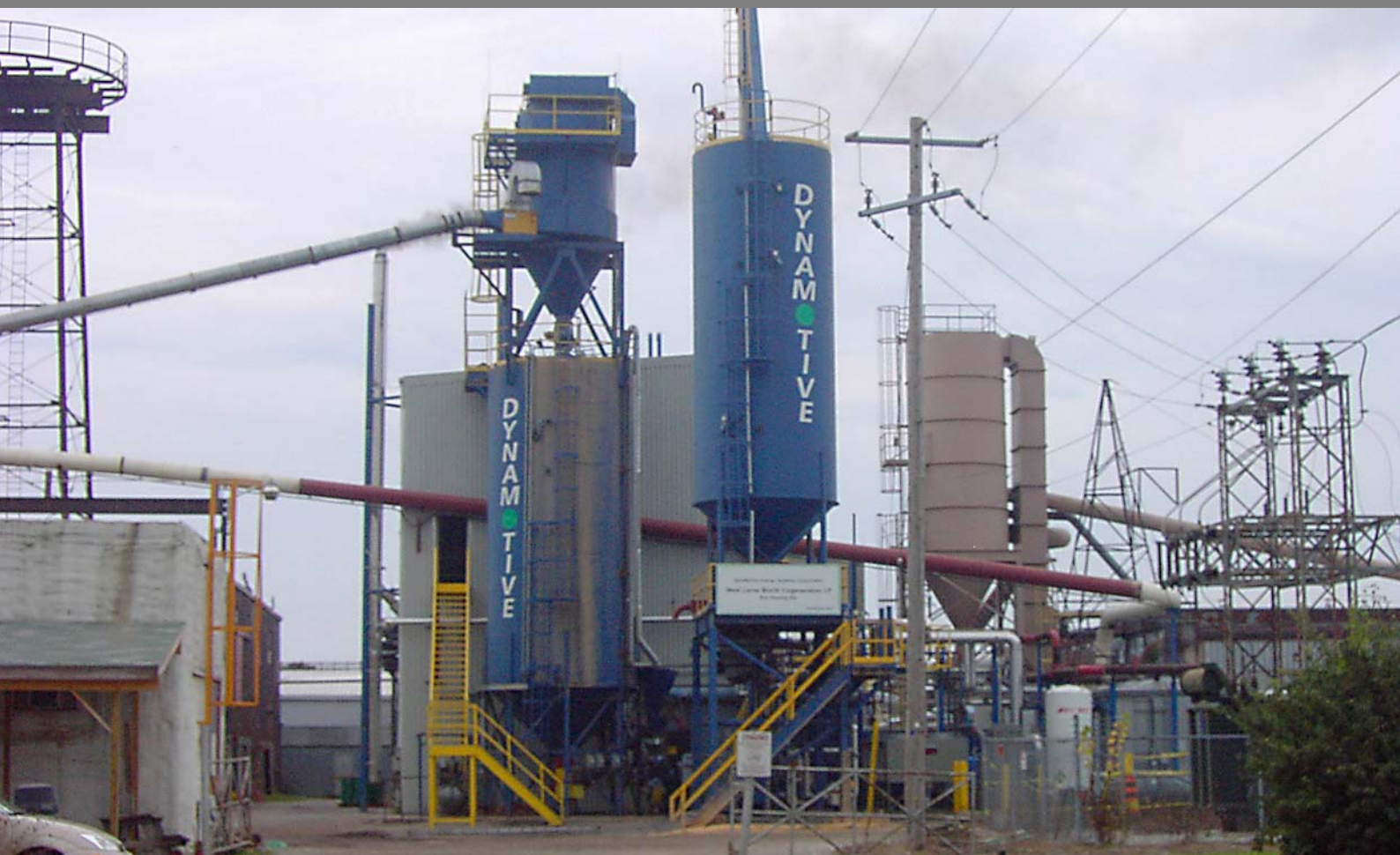
BIO OIL PRODUCTION PLANT UPGRADE - WEST LORNE - ONTARIO, CANADA – DYNAMOTIVE
